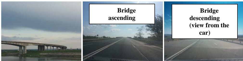
Figure 5. The bridge travelled by the vehicle
