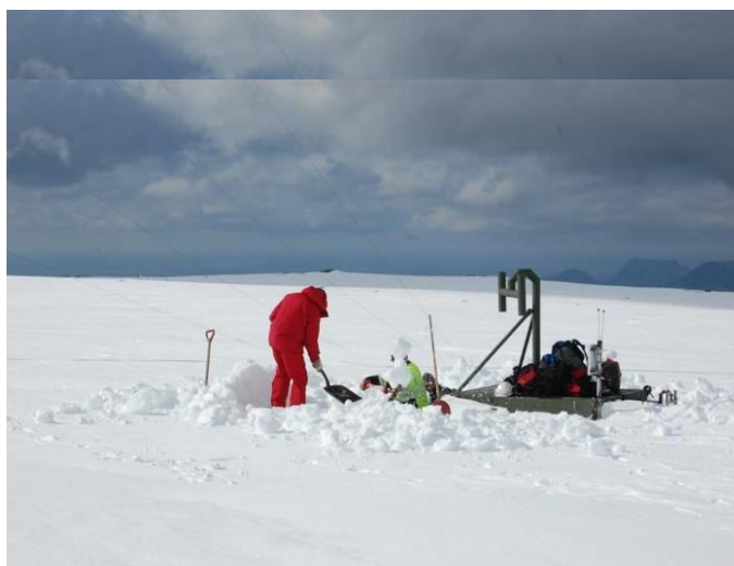
Figure 4-7: Accessing a power system in a remote location. The entire 2.5-meter high container, apart from the air inlet to the engine, has been buried. Photo credit: Lars Tallhaug, Norway
