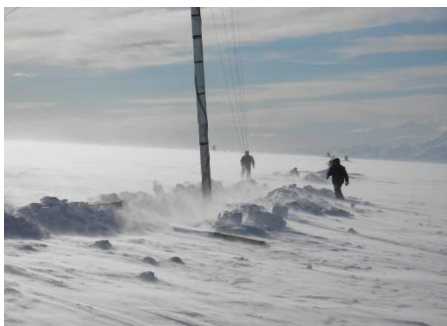
Figure 4-8: Winter meteorological tower installation in Alaska. Photo: Doug Vought, USA
