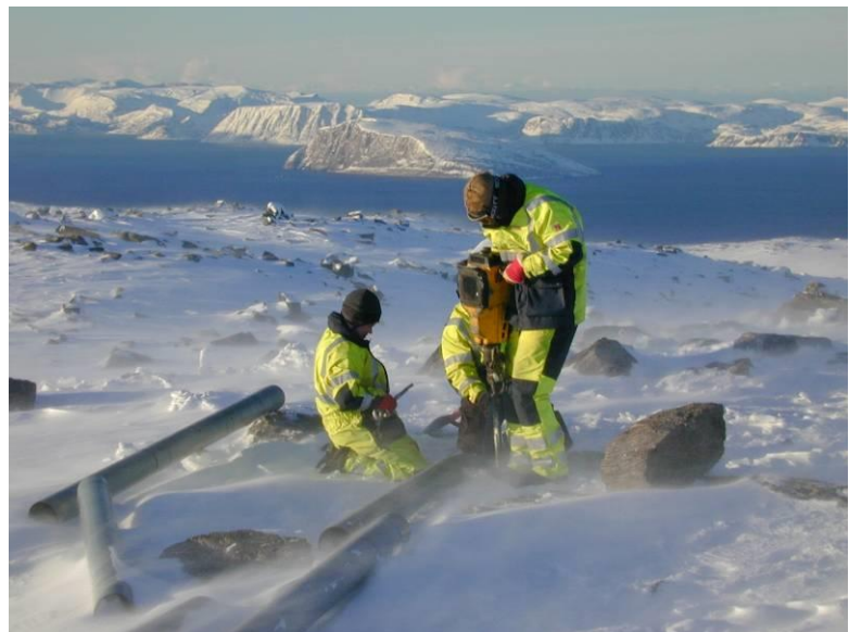
Figure 8-3: Work in extreme and cold climates requires special equipment, increased focus on personnel safety and expanded planning. Photo credit: Lars Tallhaug, Norway
